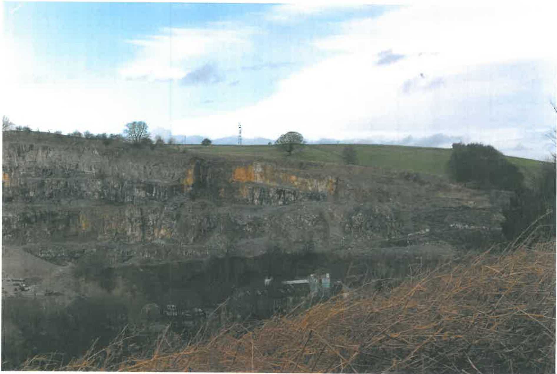
Backdale Quarry Viewpoint A (1): Looking north east towards eastern spoil tip from Bank Wood public footpath
